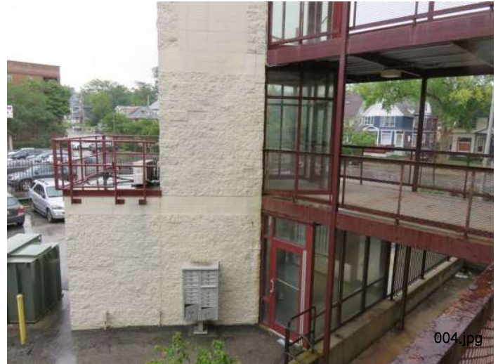
Photo: 4 Elevator core, lobby and walkway
