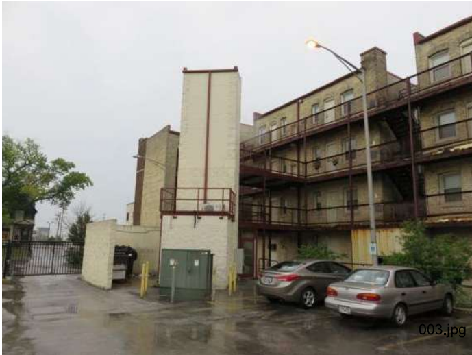
Photo: 3 Overview of elevator core
