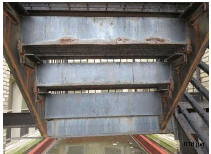
Photo: 18 Typical north stair construction
