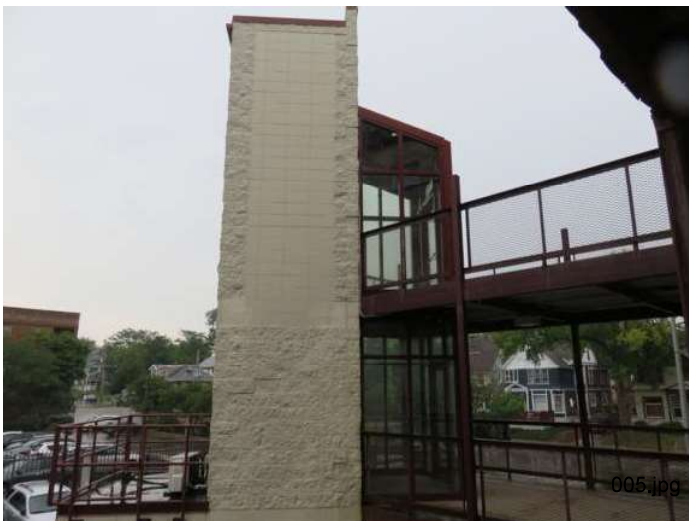
Photo: 5 Elevator core, lobby and walkway
