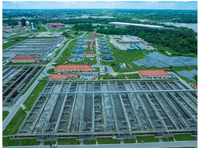
Figure 4. Back River WWTP
