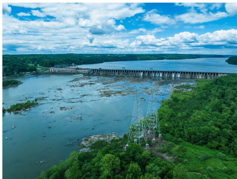
Figure 2. Conowingo Dam Source: John Roche, PTAP Aerial
