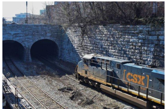
Figure 4. Howard Street Tunnel Source: Port of Baltimore
