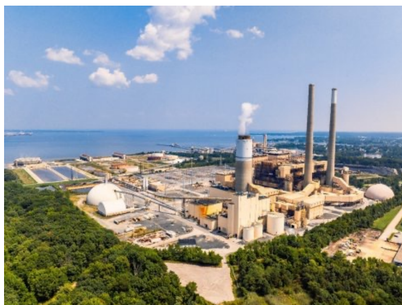
Figure 2. Brandon Shores generating station Source: John Roche, PTAP Aerial
