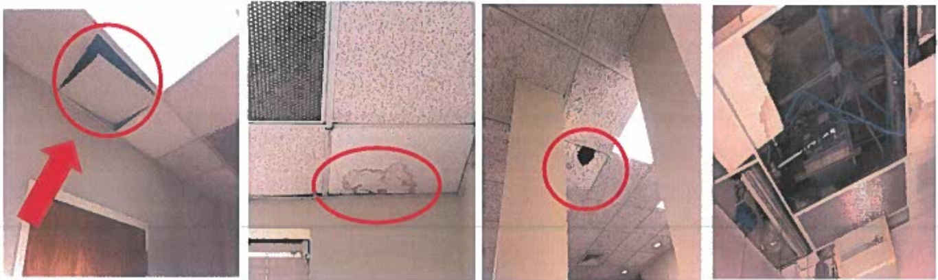
Figure 4: Unsecured and damaged access door
