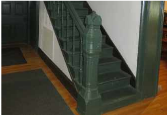
Newel post and balustrade at south foyer staircase.
