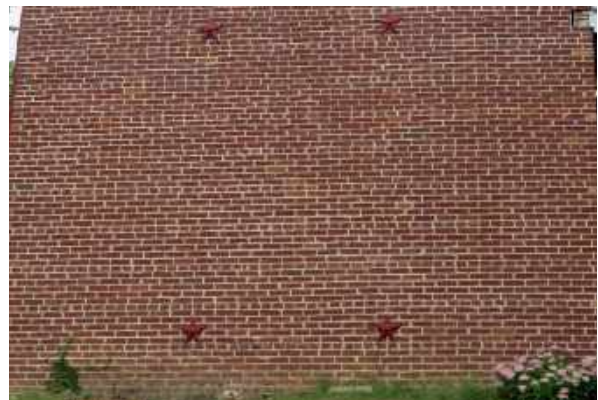
Common bond at south elevation.
