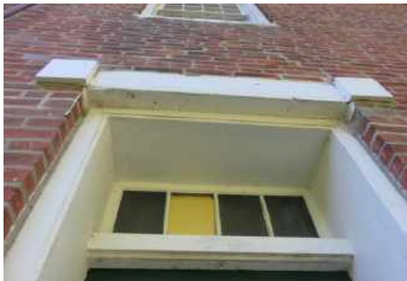
Transom with opaque replacement glass at the northwest door.
