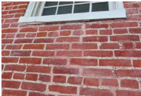
Area of repointing that does not match the rest of the masonry. Note the traces of red coating on the masonry on the right side.
