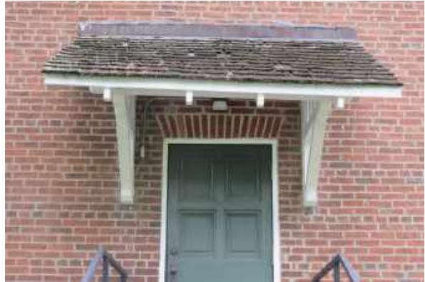
Sagging awning at the northwest entrance. Note the failed sealant at the flashing above the awning.
