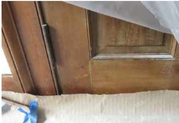
Water damaged finish at door to the north elevation in the first floor west room.
