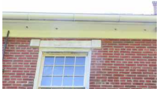
Painted over vents at the soffit underside.
