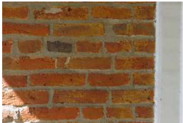
Brick with traces of yellow coating.
