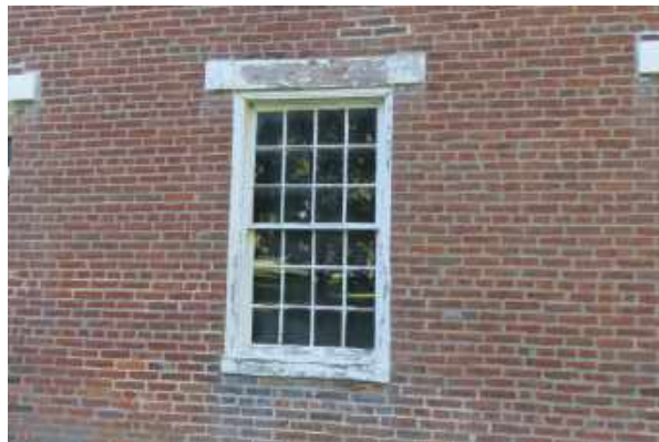
Window with heavy paint and glazing putty deterioration. This window does not appear to have been included in the 2016 scope.
