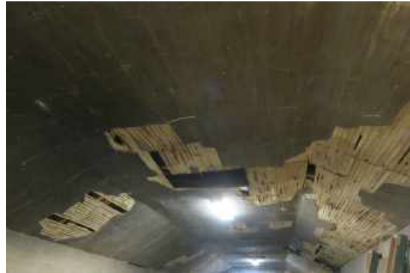
Plaster ceiling at the attic. Note staining and large areas of missing plaster and missing lath.
