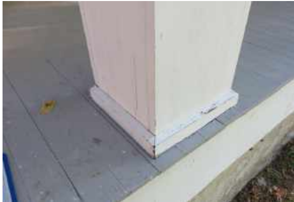
Paint deterioration, checking, and open seams in wood trim at column bases.
