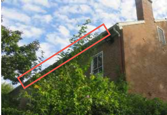
Area of damaged gutter outlined in red. Note you one can see the edges of the shingles due to the bent gutter.
