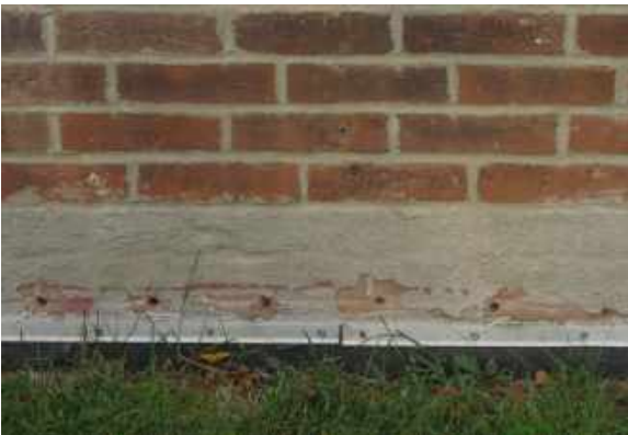
Cement parging and abandoned anchor holes above waterproofing membrane at the east elevation.
