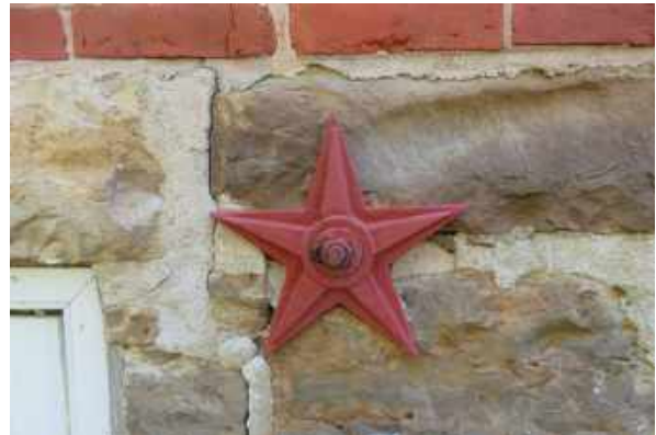
Paint deterioration and rust at building tie.
