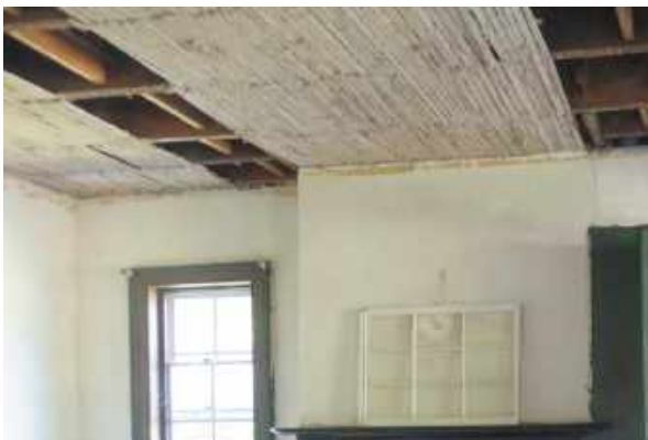
West Building. Missing ceiling in the first floor west room. Note the ghosting from a crown molding.
