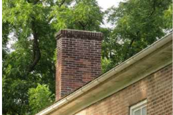
Heavily weathered and cracked mortar cap on the southeast chimney. This condition is typical of the other chimneys as well.
