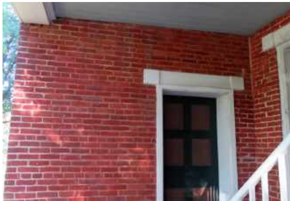
Masonry. Note the red coating on the brick, which has worn off most of the mortar joints.
