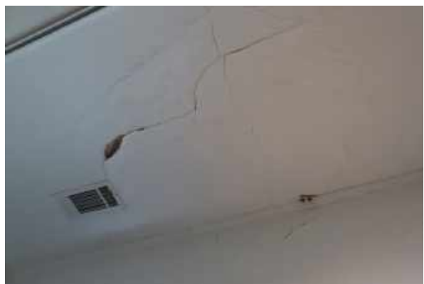
East Building. Water damaged ceiling and wall in southeast room at the second floor.
