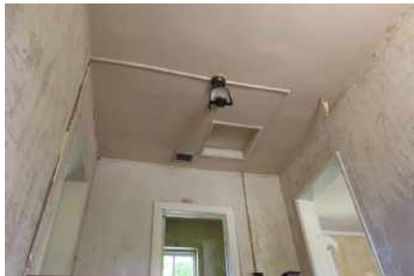
Wallboard ceiling at the second floor landing. Note the surface mounted conduit. The east and west walls of the foyer and stair are solid masonry with no room wiring behind the plaster.
