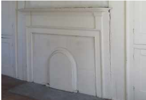
First floor east room fireplace and mantel. Note the separation at the right side.
