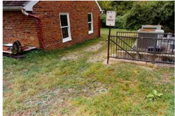
Area with thin gravel cover. Piping from the downspout in this corner can be seen through gravel in some areas.
