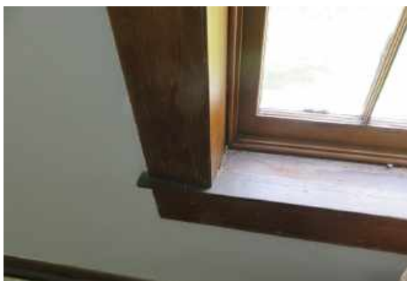
Water damaged finish at window sill from previous water infiltration issue.
