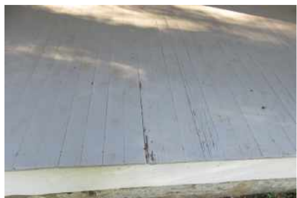
Damage and deterioration at tongue and groove floor at the first floor.
