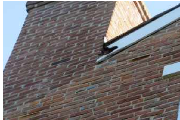
Hole in fascia panel on west elevation.
