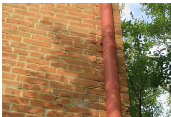
Open joints behind downspout at northeast corner.
