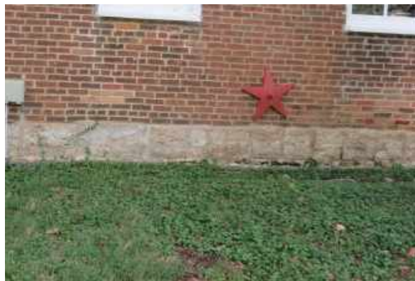
Open joints and plants growing in the gaps of the stone foundation.
