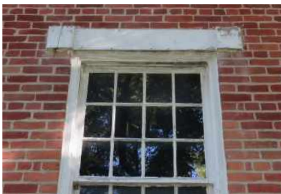
Paint and wood deterioration at flat lintel and raised wood block detail.
