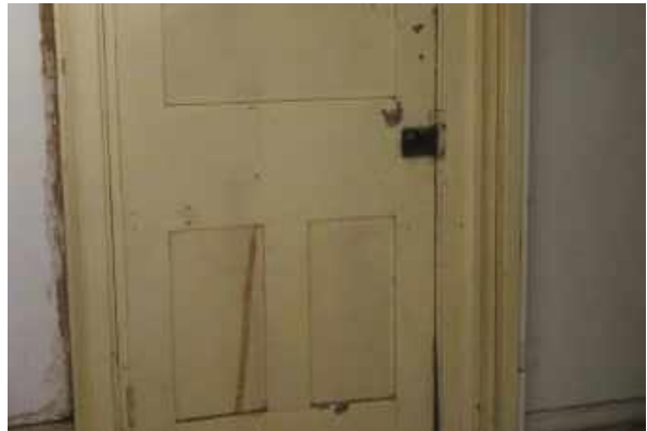
Old box lock on the porch door. Note the repaired wood check in the lower left panel.
