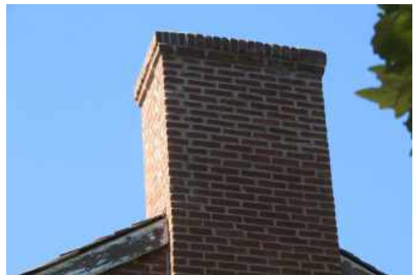
Open joints at east chimney. Note deteriorated paint at fascia panels.
