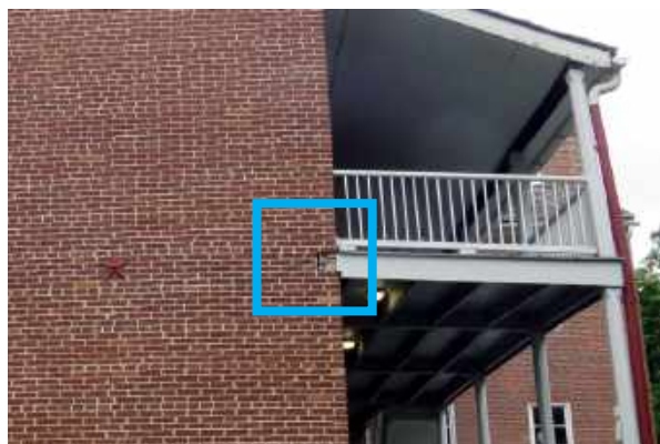
Exposed joist pocket, outlined in blue.
