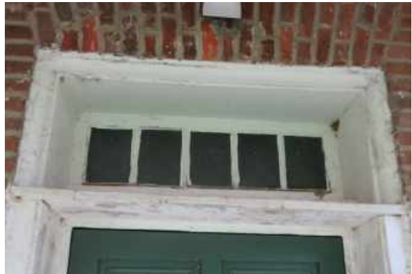
Deteriorated sealant at door surround.
