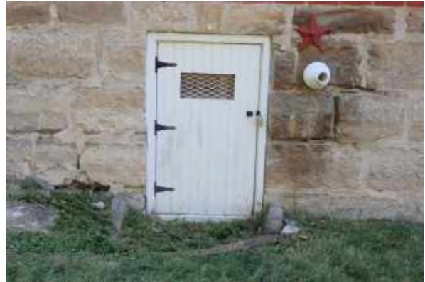
Open joint around cellar door.
