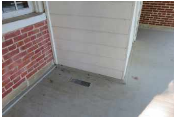
Vents to the crawl space below were added when the floor was replaced after the 1940s.
