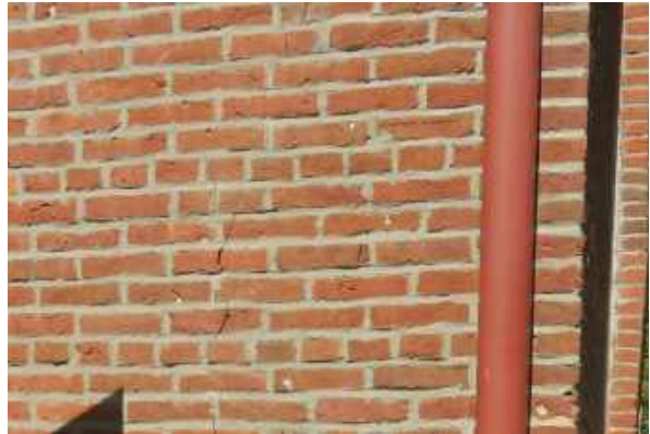
Masonry crack at southeast corner.
