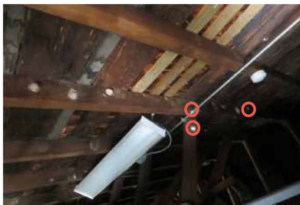
Roof from attic. Note the new sheathing boards. Spots of daylight coming through the roof are circled in red.
