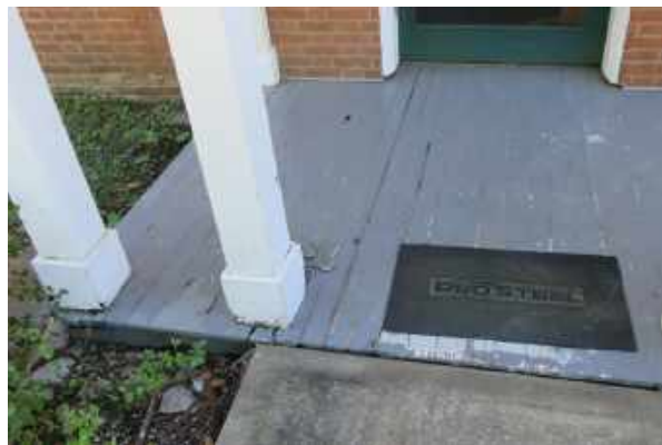
Paint and wood deterioration at north porch. Note the open seams in the column bases. These conditions are typical of both porches.
