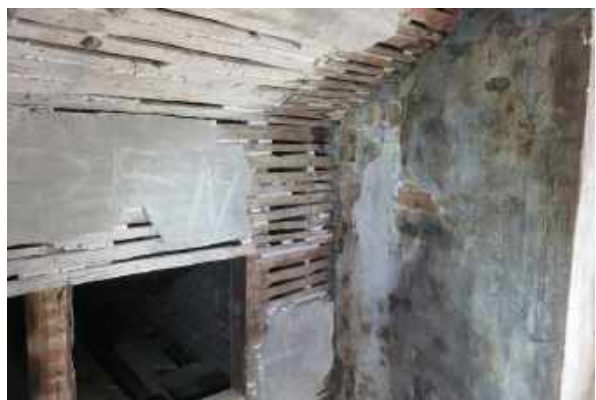
Plaster and lath in the attic at the south end. Note the graffiti scratched into the plaster on the left.
