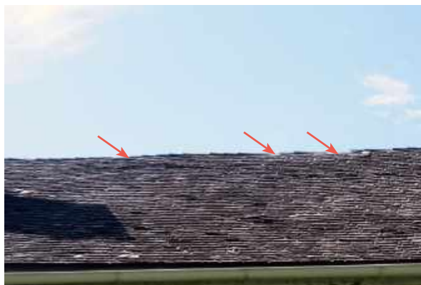
Sections of missing shingles at the ridge beam, indicated with red arrows.
