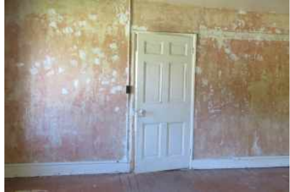
Six panel door with box lock, in the second floor west room, leading to the stair landing.
