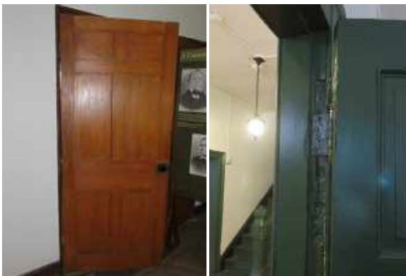
Left: six-panel door in south exhibit rooms, with box lock. Right: ghosting and damage from many different door installations at office door.
