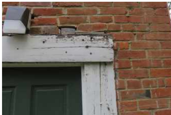
Wood and paint deterioration at kitchen door.
