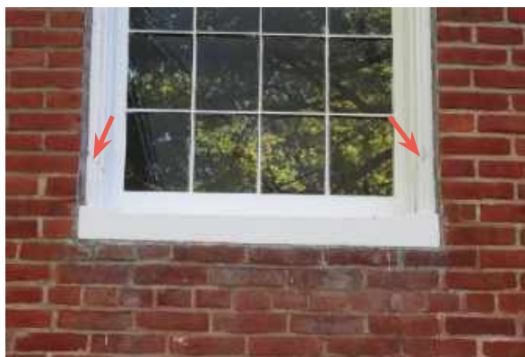
Repaired window where seams from dutchman repairs are visible through the paint. Note the unpainted grey sealant at the edges of the window frame.
