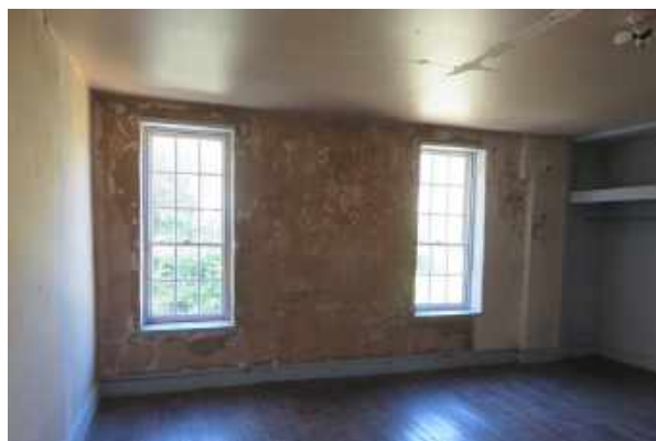
Plaster wall at second floor room in the rear addition. Note the ceiling damage and unfinished drywall on the left.
