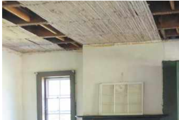
Missing ceiling in the west room. Note the ghosting from a crown molding.
