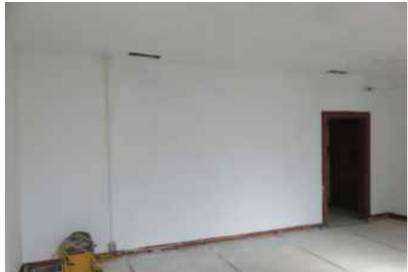
New wall at second floor west room. Note that this floor slopes to the center of the room.
