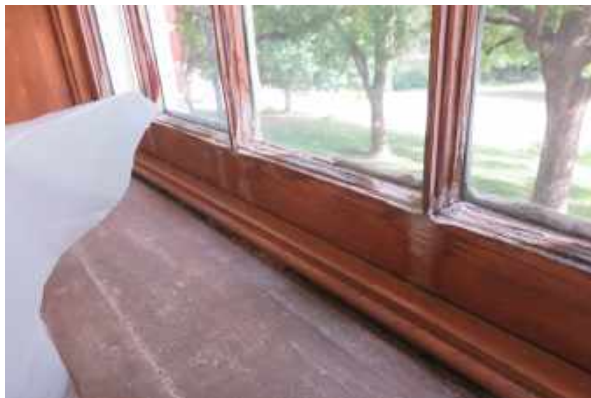
North Building. Water damage at new sash, deteriorating finish at window sill.
