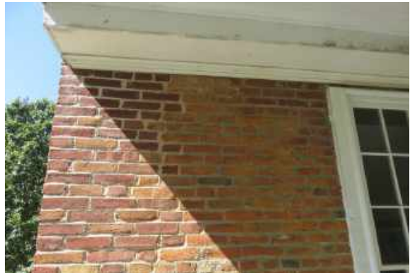
Repointing at an area of brick replacement. Note the different colors of mortar and the yellow coating on the bricks to the right.
