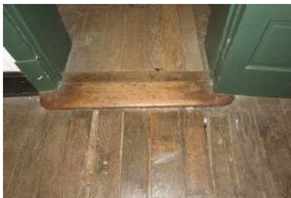
Large threshold at south door to second floor central room, due to floor slope. Note the broken board to the right.
