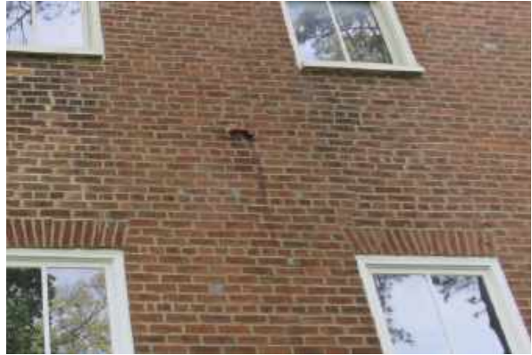
Pipe at the north end of the west elevation leaking an unknown substance down the brick.
