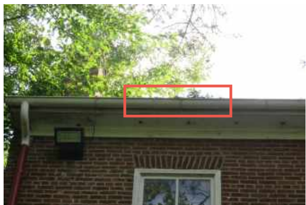
Pine needle and plant buildup in gutter visible from ground level, outlined in red.
