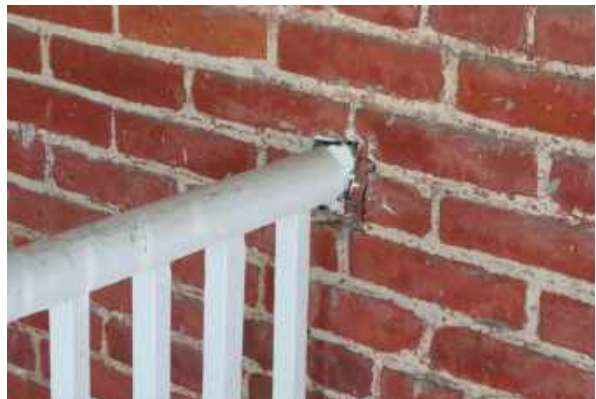
Rail termination at the masonry. Note the wood blocking added to stabilize the railing.
