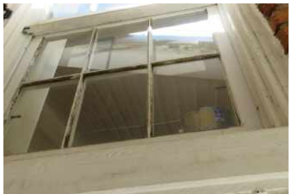
Deteriorated paint and glazing material at a window on the south elevation.
