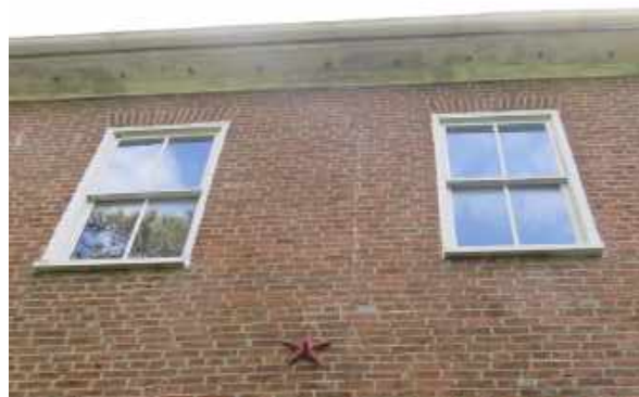
Second floor windows at the west elevation, showing signs of paint deterioration at bottom rail of upper sash.
