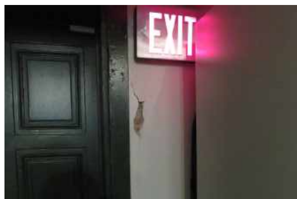
Plaster cracking at northwest door. The masonry is exposed in this area, and multiple previous finishes are visible.
