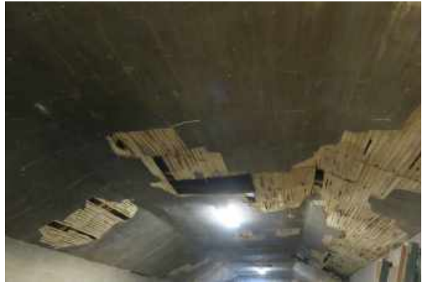
East Building. Plaster ceiling at the attic. Note staining and large areas of missing plaster and missing lath.
