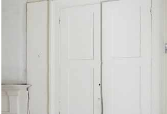
Missing and over-painted hardware on built-ins.
