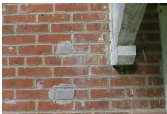
Patch executed in grey mortar.
