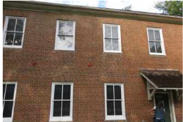
Exterior brickwork, with splayed lintels over windows.
