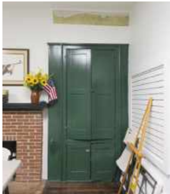
Conference room built-in. Note the paint reveal showing stenciling above the cabinet.
