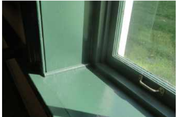
Windows on the first floor did not open and appear to be painted shut. It is unclear if this was intentional or due to high temps and humidity during the site visit.
