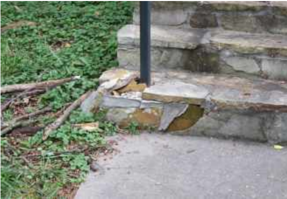
Damaged corner of northwest stair. Note that this area has been repaired, but that repair has failed.
