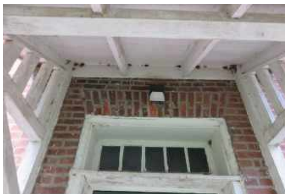
Deteriorated paint and insect nests below awning. Note the overpaint and deteriorated paint at the door surround.
