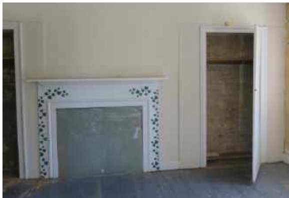
Covered fireplace in second floor east room. Note that the built-ins may have been converted to closets relatively early, as this is a mortis and tenon panel door, not a modern hollow door.
