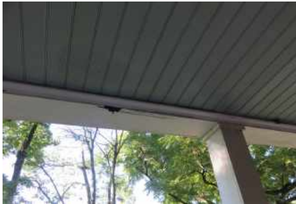
Wood deterioration at porch soffit.
