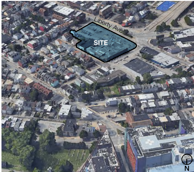
Aerial view from North
