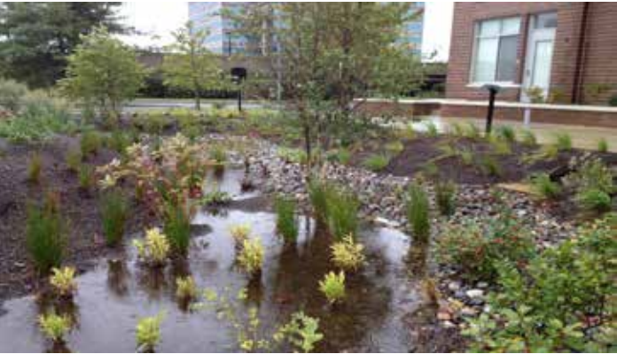
Rain Gardens - Natural depression in the landscape help capture, store, cleanse and infiltrate stormwater.
