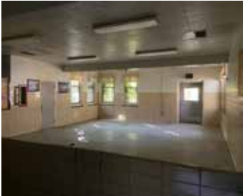
Meyer Building | Credit: EHT
