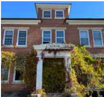
“B” Building | Credit: DCI
