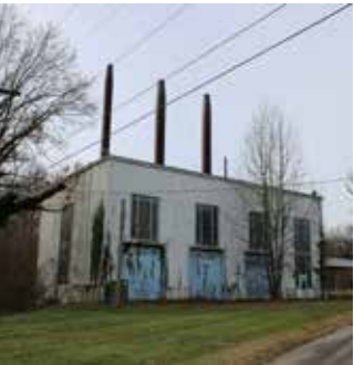
Boiler Plant | Credit: EHT
