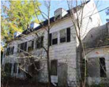
Superintendent's House | EHT
