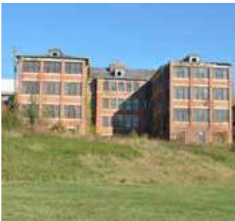
Laundry Building | Credit: DCI
