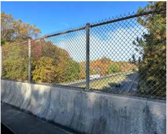
Bridge over I-97 - source: Design Collective
