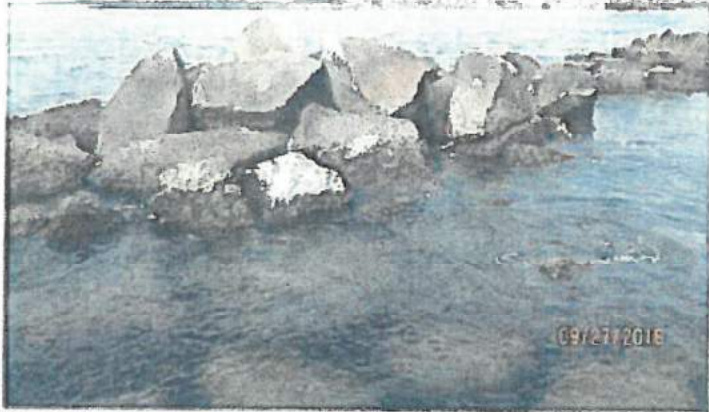
Fig. 19. View from estimated angle of impact. Boulder with most white transfer is initial impact point.
