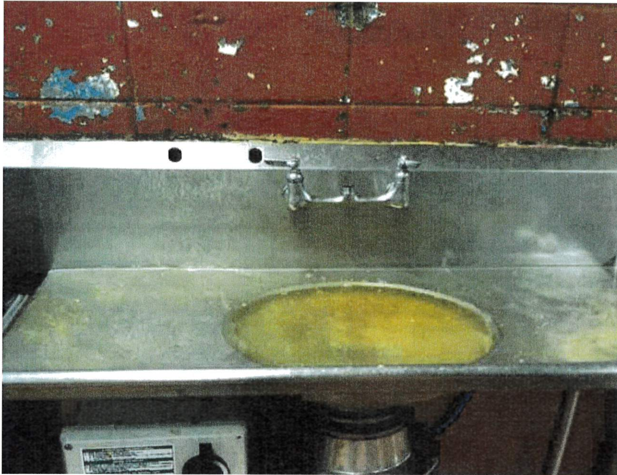
A June 2019 Mississippi Health Department inspection at the Mississippi State Penitentiary at Parchman shows a clogged sink with an inoperable garbage disposal. Mississippi Health Department
