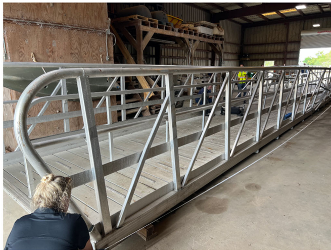
Subject Crescent gangway with flimsy top chord and insufficient structural members
