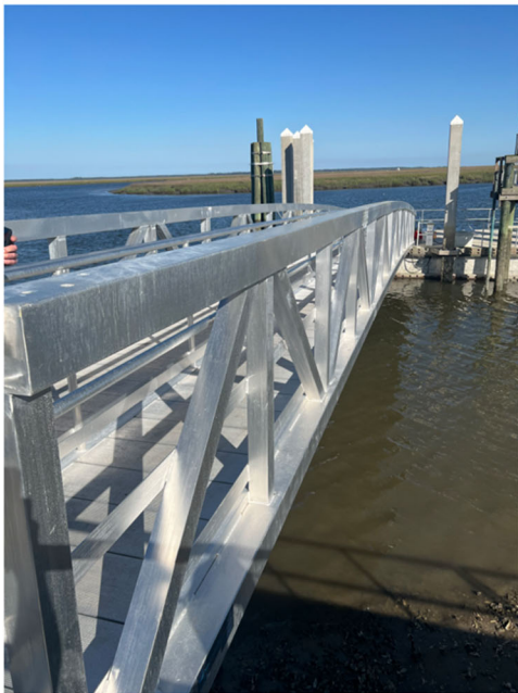
New Meridian gangway with industry standard top chord and robust structural members
